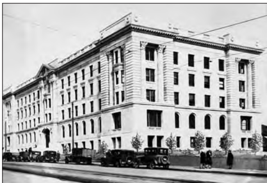
The Bowker Building in 1931. (PAA BL67)
