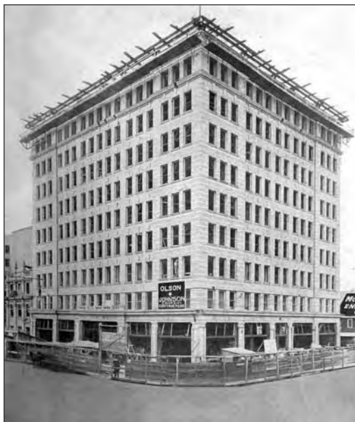
The McLeod Block, one of Edmonton's first skyscrapers, c. 1915. (Edmonton: Alberta's Capital City - 1914 at CEA)
