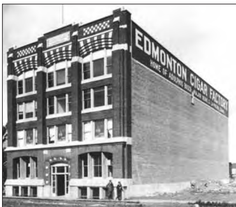
The H.V. Shaw cigar factory and warehouse, 1921. (GAI NA-1328-66444)
