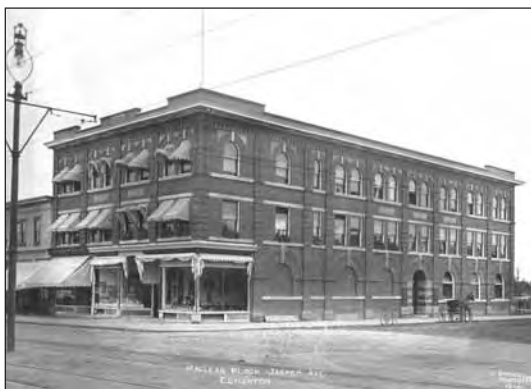
The MacLean Block one year after its construction, 1910. (PAA B4228)
