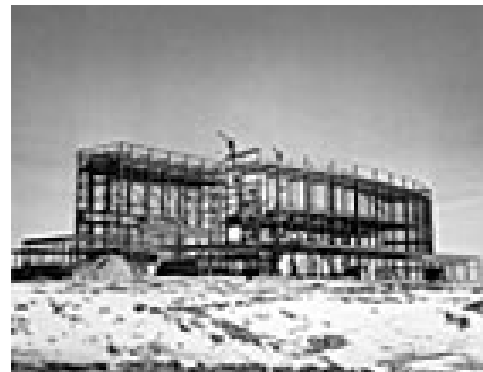
Northern Alberta Jubilee Auditorium, Under Construction, Edmonton, AB
